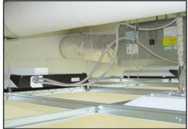
Limited Access Working Space
