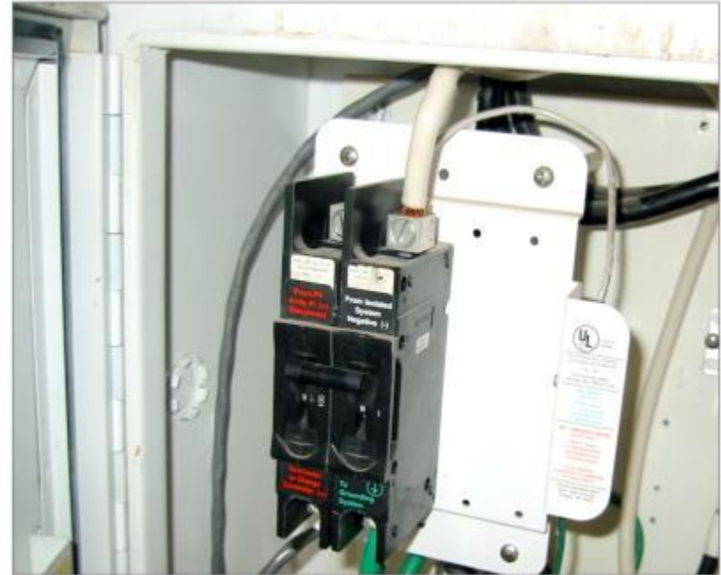
690.41(B) (GFP) Ground-Fault Protection
